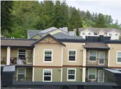
Our understanding is that the exterior was last painted in 2014 with an 10 year product. We found this consistent with the current condition and have budgeted for the next paint cycle in 2024. There have been several improvements in exterior paint the last few years and we have found that the use of a high quality paint of an eggshell or comparable sheen and biennial paint touchup can increase the paint life span considerably and reduce overall maintenance costs.
