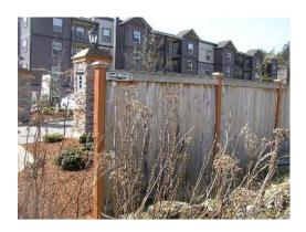
We found the wood fence to be in fair to good condition. Wood fences in the northwest can be expected to provide a useful life of 15 years if kept in good condition and coated with a high quality wood preservative on a regular basis.
