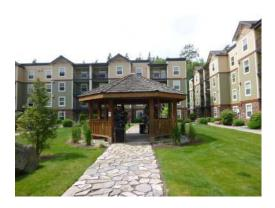
The gazebo appears to be in good condition and should not require any near term repairs. We have included a budget for future repair and the evetual roof material replacement.
