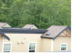
Each of the three main buildings include several sections of shingled roofing material. The gables and sloped portions at the main roof level and the entrances on the ground floors. This material appears to be a 30 year shingle as manufactured by Pabco or similar. The shingles appear to be in good condition, however we did notice several areas where moss has grown and should be removed. We recommend a close inspection and application of a quality moss retardant to control future growth.
