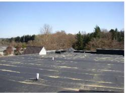
All of the roof sections appear to be in good condition and in line with the age following replacement. To maximize the useful life it is recommended that annual inspections be conducted and any damage found be corrected immediately. Cleaning should very gentle and only be carried out by knowledgeable professionals.
